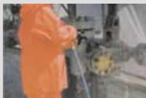
Fig. C: Removal of existing coating by pressure washing at 17 MPa
