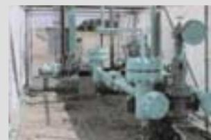
Fig. D: Complete project after application of 50-75  $\mu\text{m}$  DFT of aliphatic urethane topcoat
