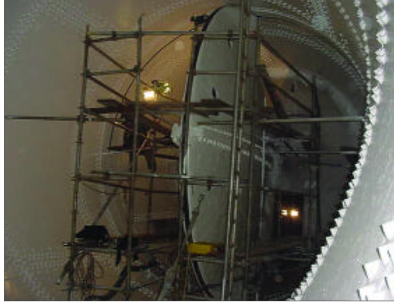
*Penstock at generator station where modified phenalkamine was applied for rapid immersion service
