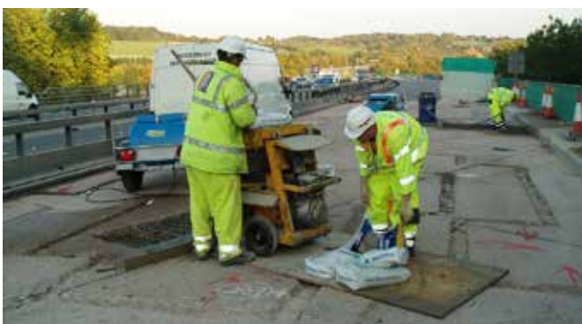
Intercrete 4802 sets 10 minutes, achieving a final strength of over 60MPa
