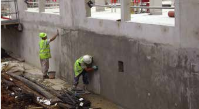
Intercrete 4822 colours can be blended to match the shade of concrete
